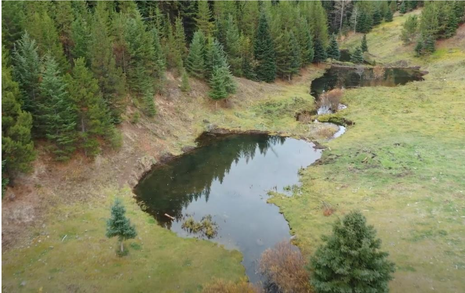
Ponds formed by artificial beaver dams (BDAs) along Howarth Creek, B.C. These structures were built in 2021.
