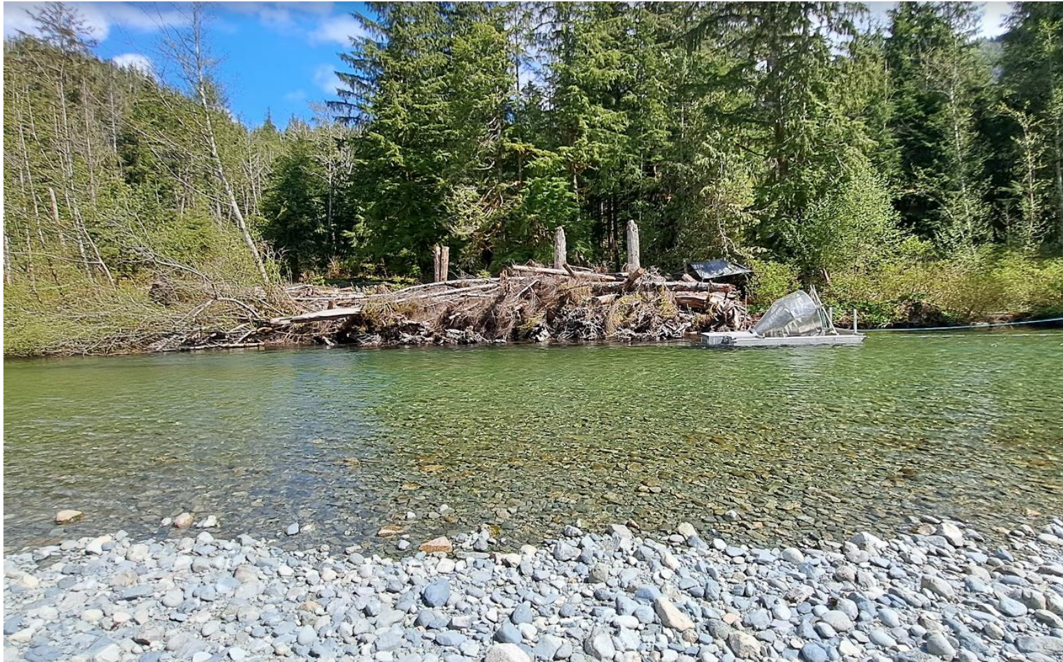
Constructed Logjam on the Bank of Tranquil River
